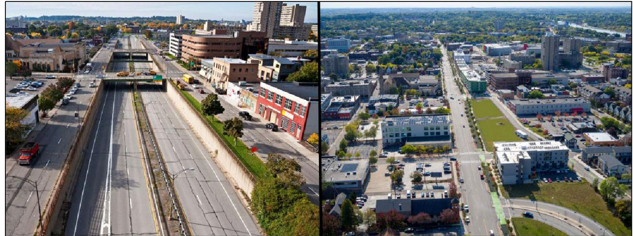
Inner Loop Expressway (East) – Rochester, New York (2014-2017)
