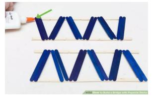
3. Glue cradle supports to the top of your bridge and glue upper support beams.
