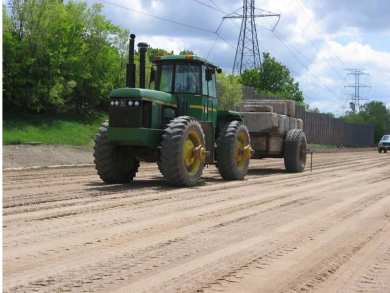
Figure 1.3. Test rolling a compacted subgrade.
