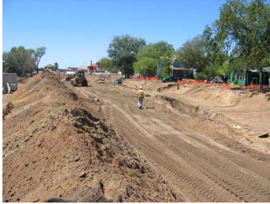
Figure 2.1. Construction of Highway 10 in Staples, MN.
